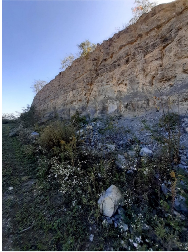
Photo 3 Close up of the highwall seen in Photo No.1.
